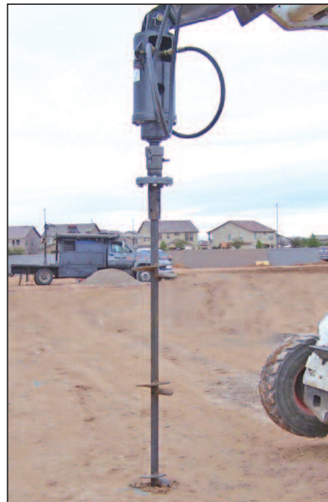
Typical MB Brace Badger Installation
